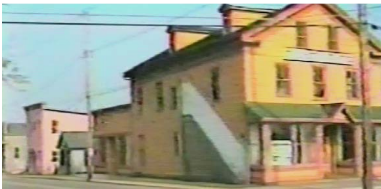
This photo shows the building after the enclosed stairway had been removed but before new windows were installed on the south side.
